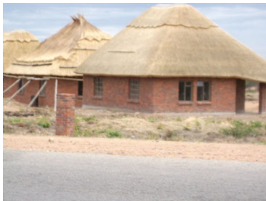
( A LODGE STILL IN CONSTRUCTION)
